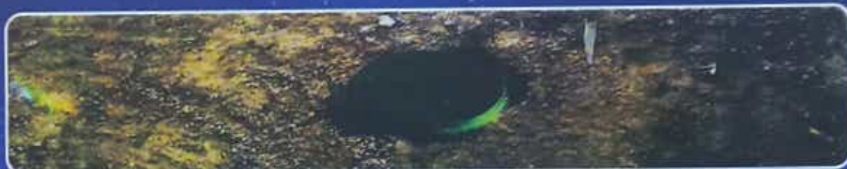
Step 7. Cover the AE Power Earthing Cover with soil and ram properly
